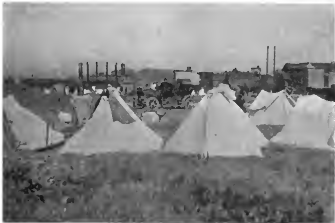
CAMP-GROUND FOR DESTITUTE EARTHQUAKE VICTIMS.
